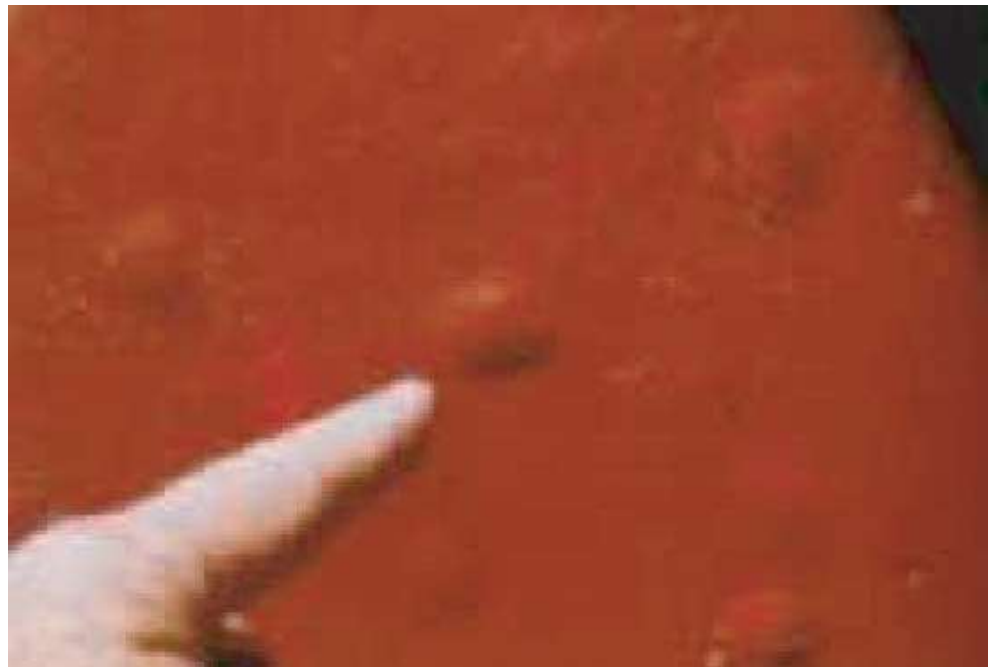
Figure 6.6.14 Blistering on a Laminated Surface
