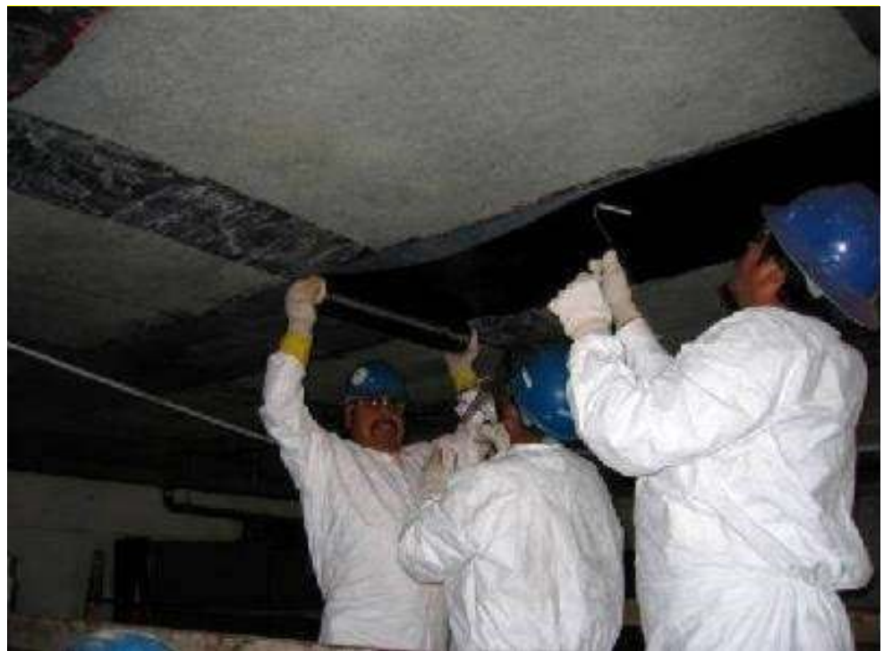
Figure 6.6.1 Concrete Beam Repaired Using FRP
