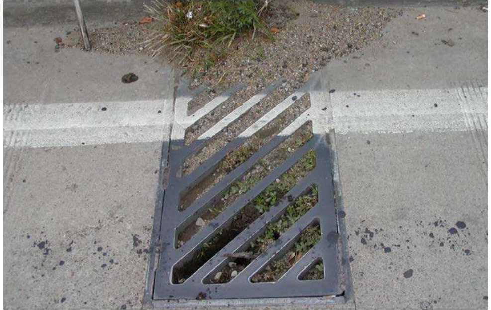
Figure 7.5.30 Clogged Scupper
