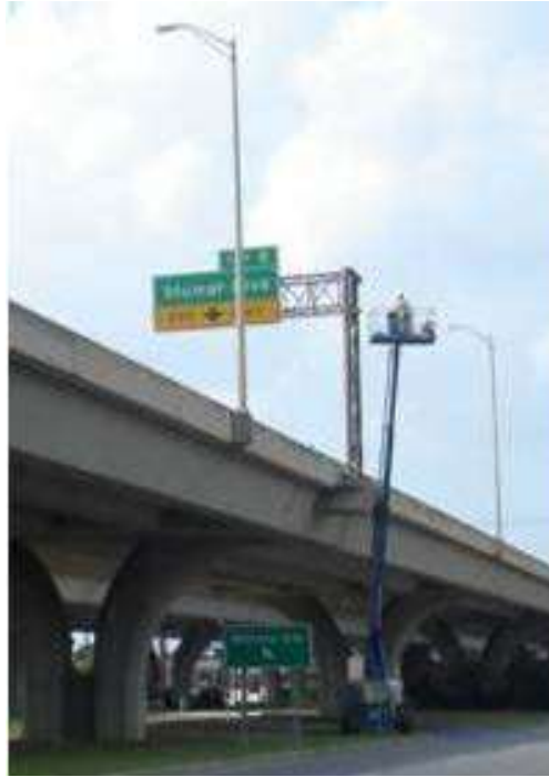
Figure 7.5.33 Sign and Light Structures Attached to a Bridge
