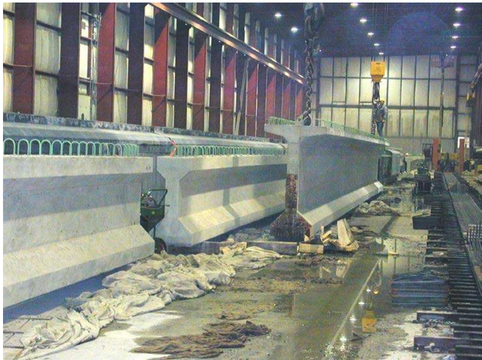
Figure 7.2.4 Prestressed Concrete Beams with Shear Connectors Protruding for Composite Deck
