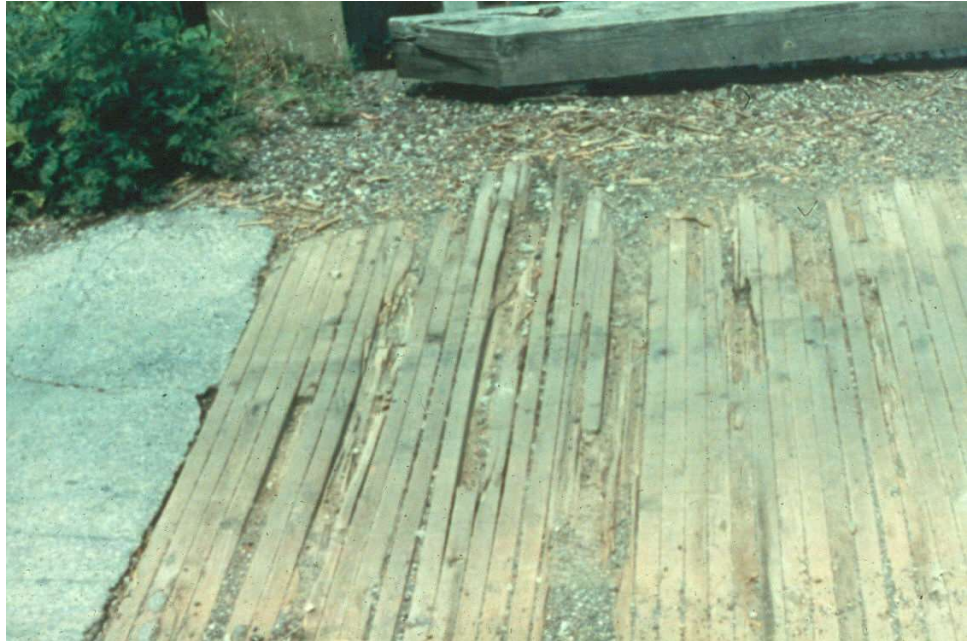
Figure 7.1.8 Wear and Weathering on a Timber Deck
