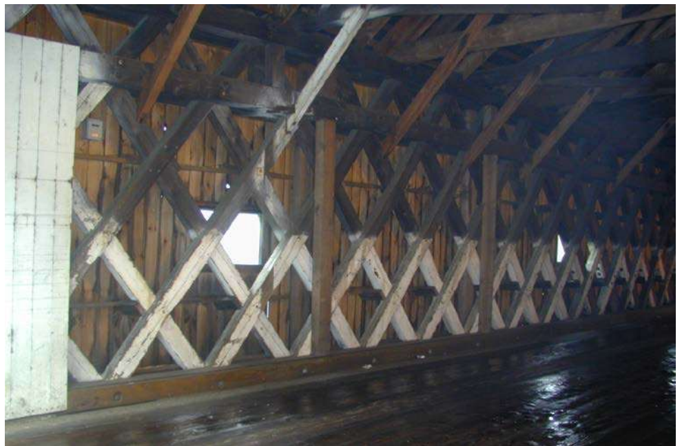
Figure 8.1.10 Town Truss Design
