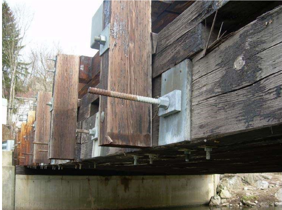
Figure 7.1.4 Stressed-laminated Deck
