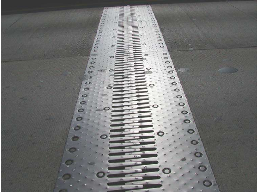
Figure 7.5.14 Finger Plate Joint
