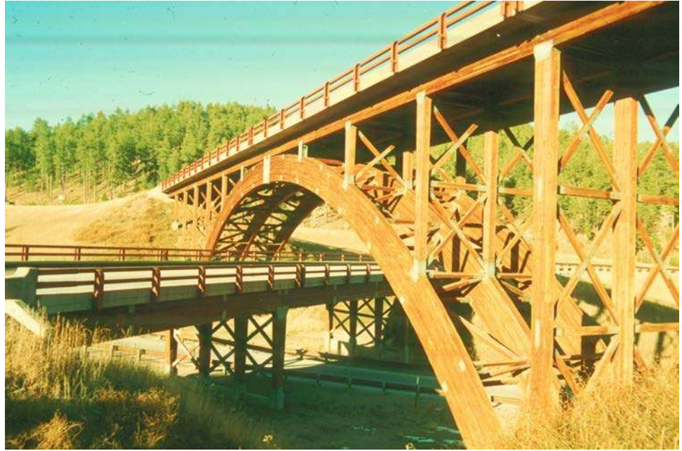
Figure 8.2.6 Glulam Arch Bridge over Glulam Multi-beam Bridge (Keystone Wye interchange, South Dakota)
