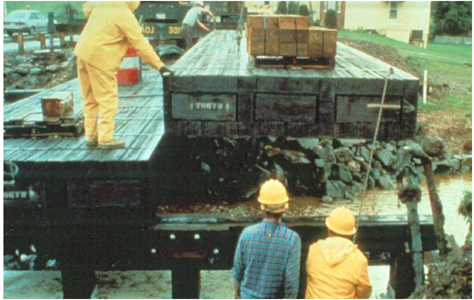
Figure 7.1.5 Structural Composite Lumber Deck Using Box Sections
