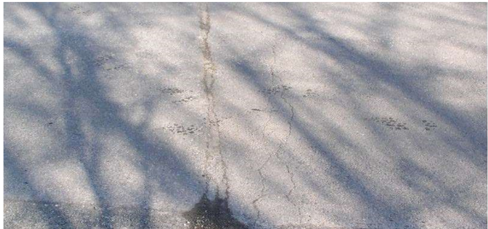
Figure 7.5.28 Asphalt Wearing Surface over an Expansion Joint
