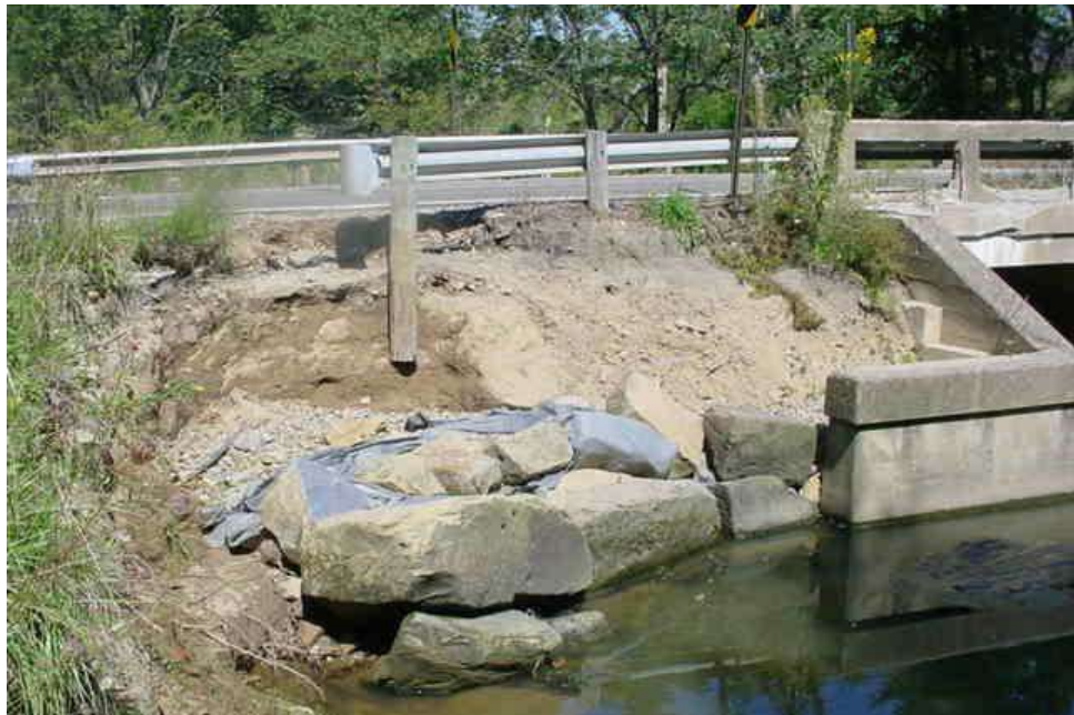
Figure 7.6.14 Erosion Reducing Post Embedment
