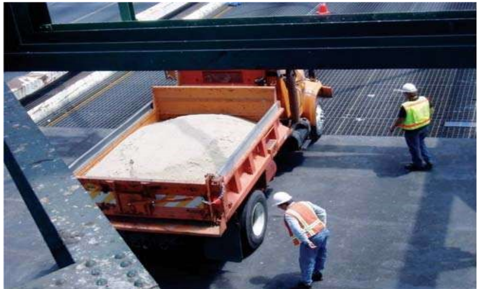
Figure 7.3.5 Use of Truck for Visual Inspection of FRP Deck
