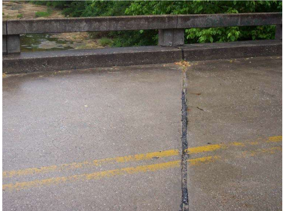
Figure 7.5.2 Pourable Joint Seal
