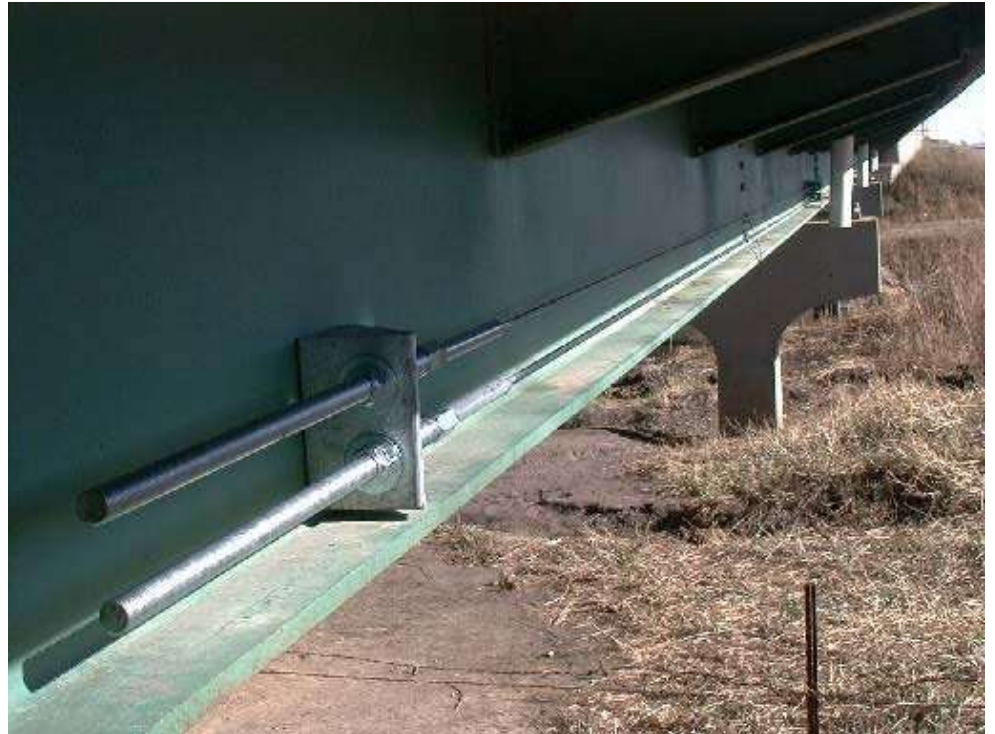
Figure 6.6.3 CFRP Post-tensioned Steel Girder
