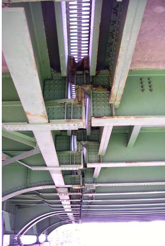
Figure 7.5.29 Support System under a Finger Plate Joint
