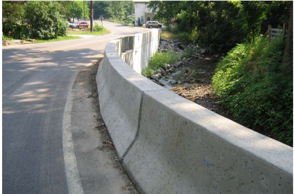
Figure 7.6.6 Acceptable Bridge Rail
