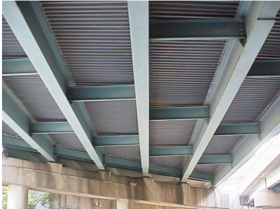
Figure 7.2.1 CIP Concrete Deck with Stay-in-Place Forms
