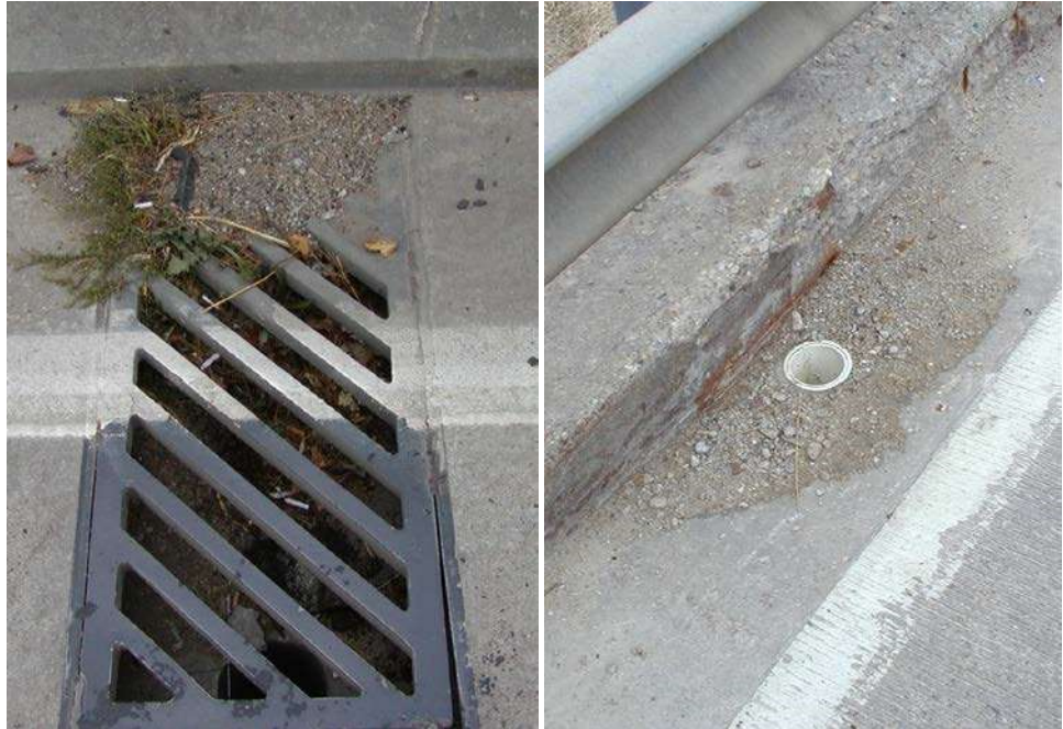
Figure 7.5.19 Bridge Deck Scupper (left) and Deck Drain (right)
