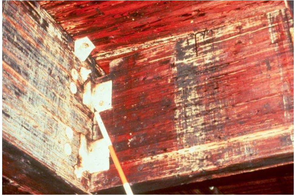
Figure 8.2.13 Typical Diaphragm for a Glulam Multi-beam Bridge
