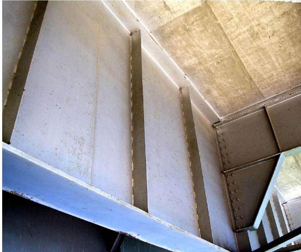
Figure 6.4.54 Intermittent or Stitch Welded Transverse Stiffeners
