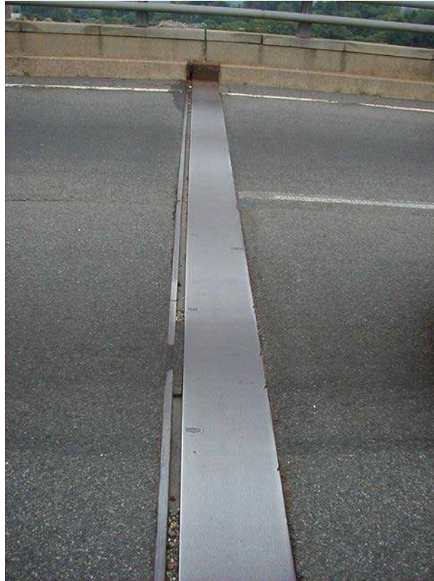
Figure 7.5.17 Sliding Plate Joint
