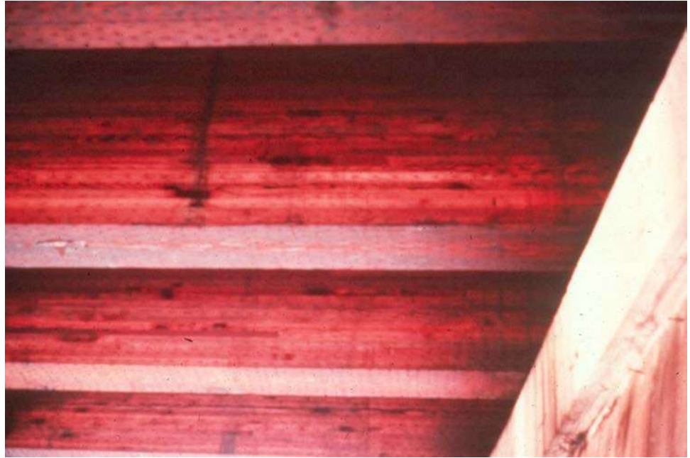
Figure 8.2.10 Close-up View of Glulam Bridge Showing Laminations
