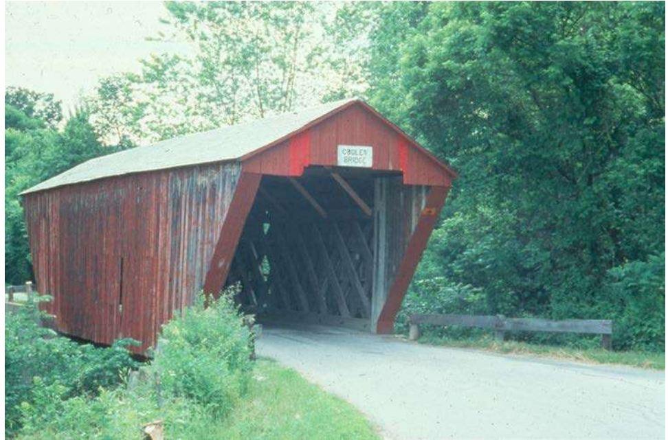
Figure 8.1.5 Town Truss Covered Bridge
