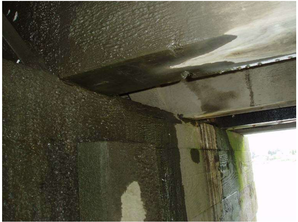
Figure 8.1.11 Bearing Area of Typical Solid Sawn Beam
