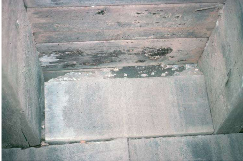
Figure 8.1.14 Typical Timber End Diaphragm
