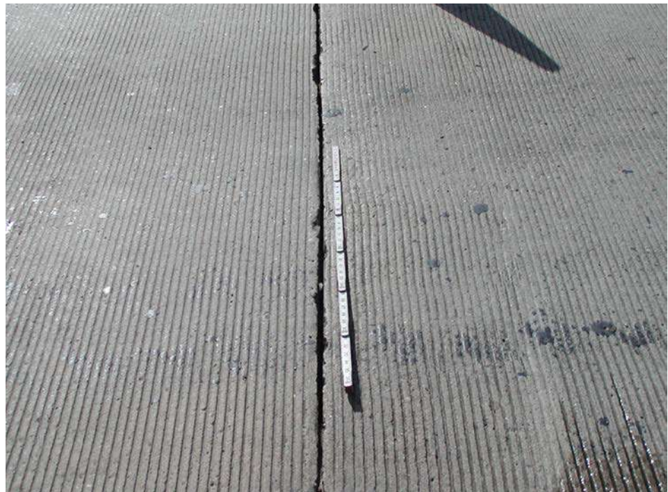
Figure 7.5.12 Open Expansion Joint
