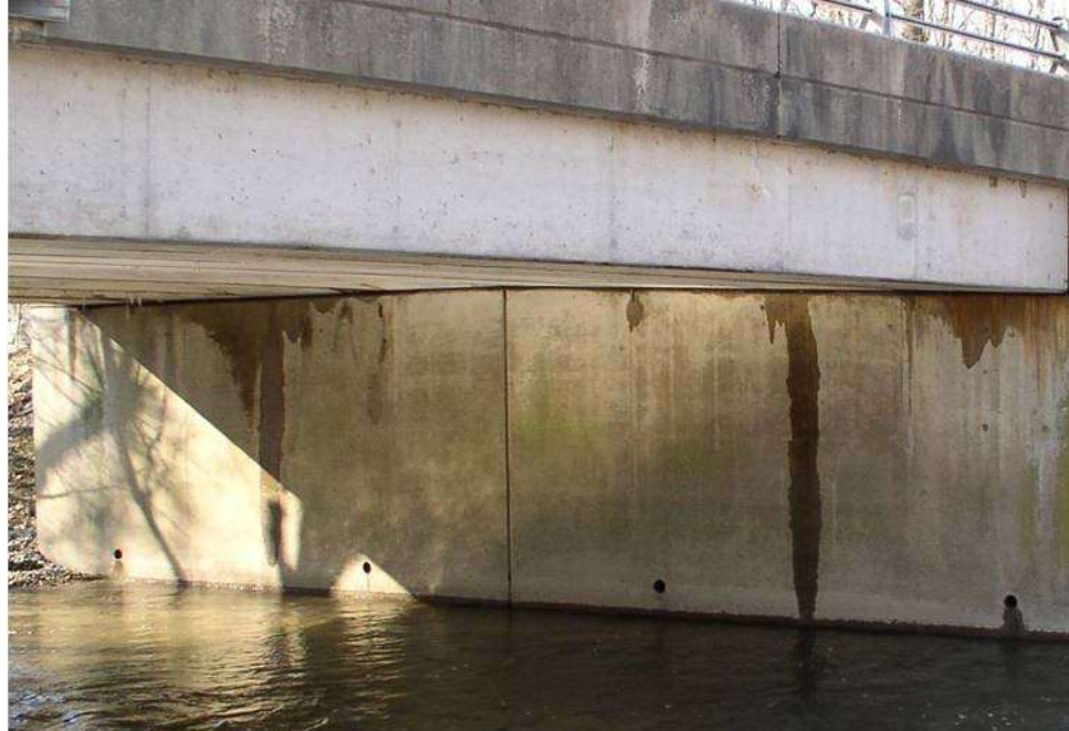
Figure 7.5.23 Weep Holes
