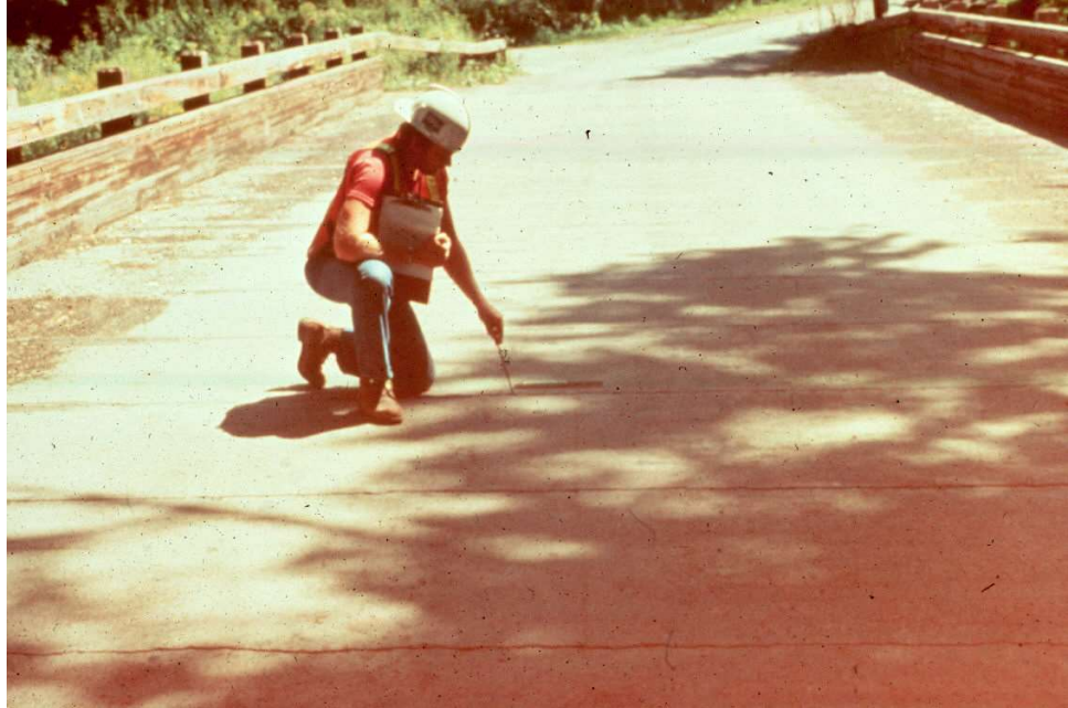
Figure 7.1.7 Inspector Probing Timber with a Pick at Reflective Cracks in the Asphalt Wearing Surface
