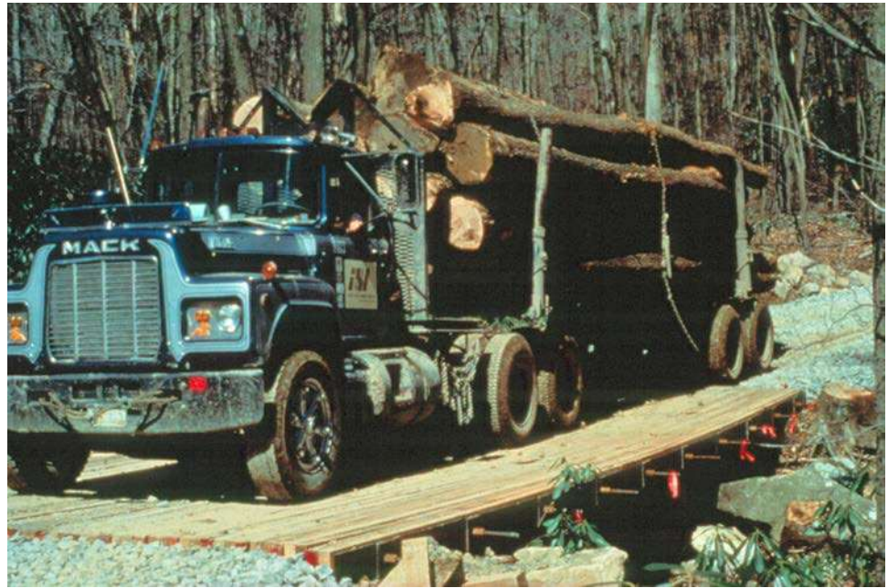
Figure 8.3.1 Stress-Laminated Timber Slab Bridge Carrying a 90,000-Pound Logging Truck (Source: Barry Dickson, West Virginia University)
