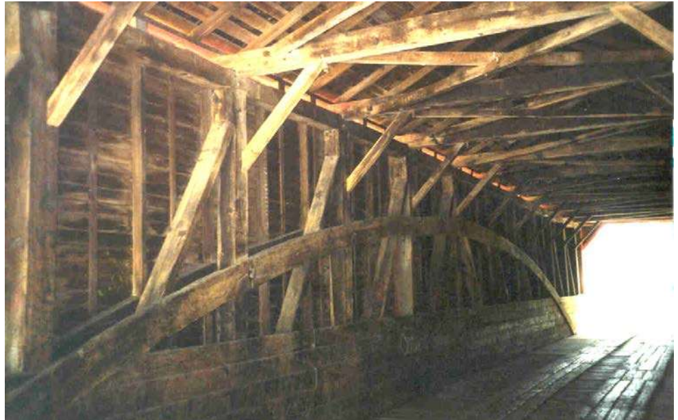
Figure 8.1.9 Inside View of Covered Bridge with Burr Arch-truss Design
