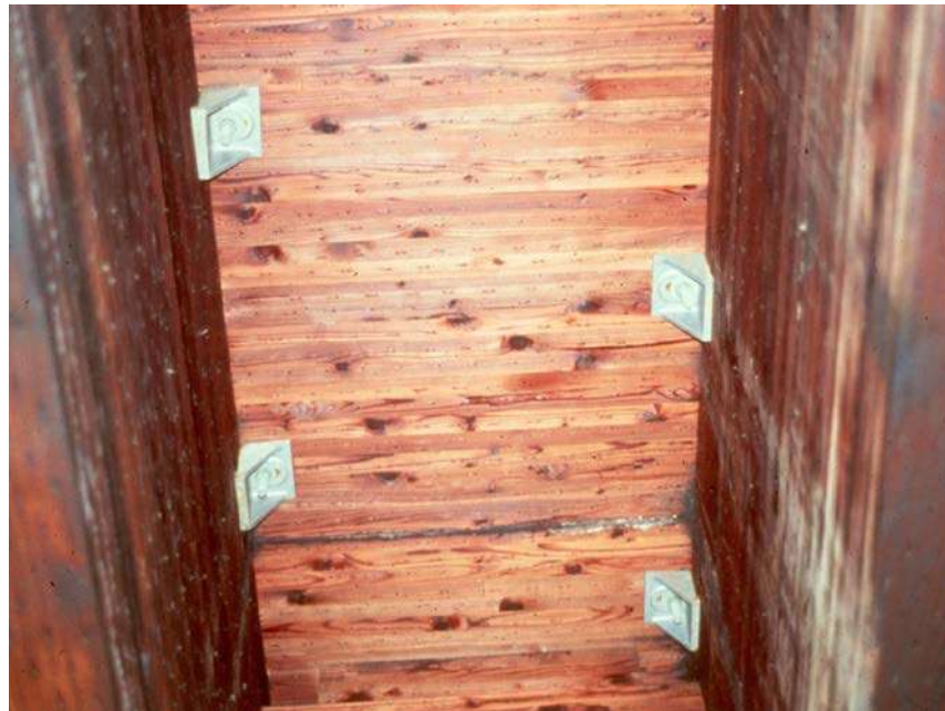
Figure 7.1.3 Glued-laminated Deck Panels Attached to Superstructure
