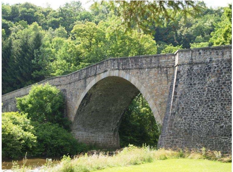
Figure 6.5.1 Stone Masonry Arch
