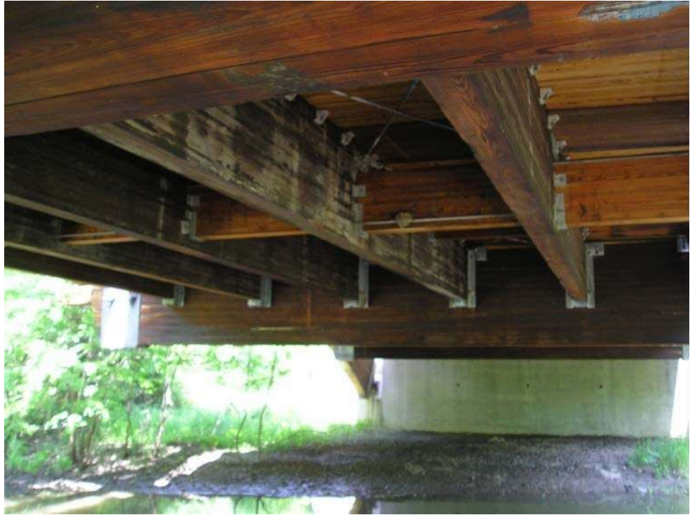
Figure 8.2.2 Underside View of a Glulam Multi-beam Bridge
