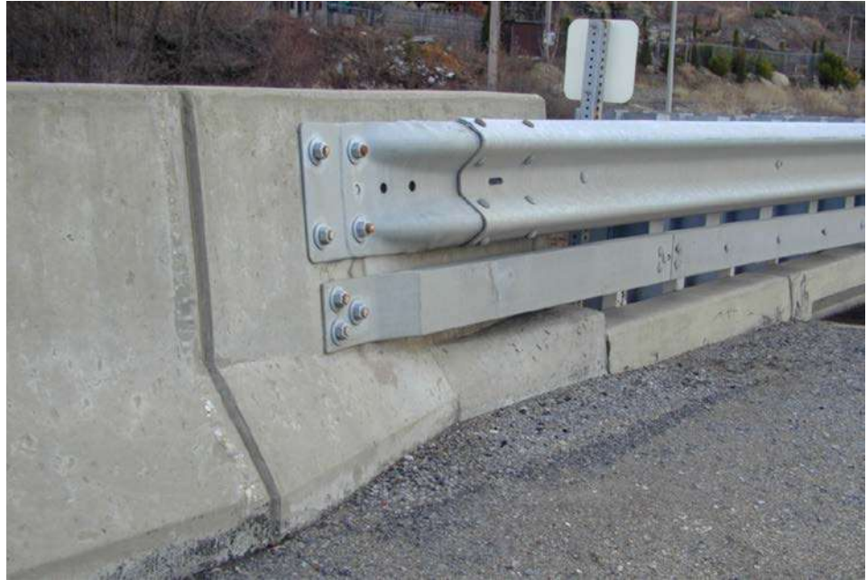
Figure 7.6.15 Proper Nesting of Guardrail at Transition
