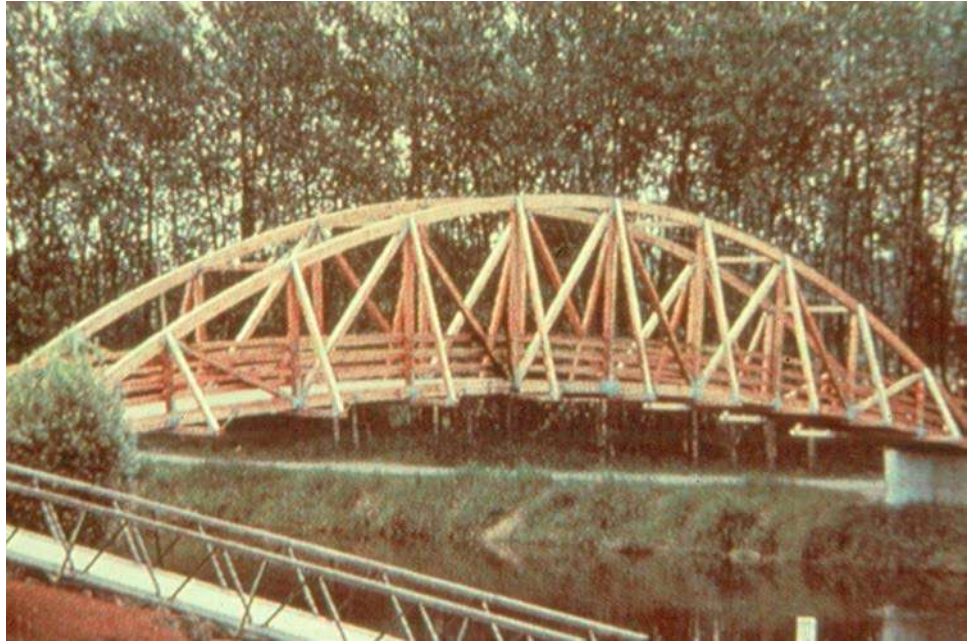
Figure 8.2.4 Bowstring Truss Pedestrian Bridge
