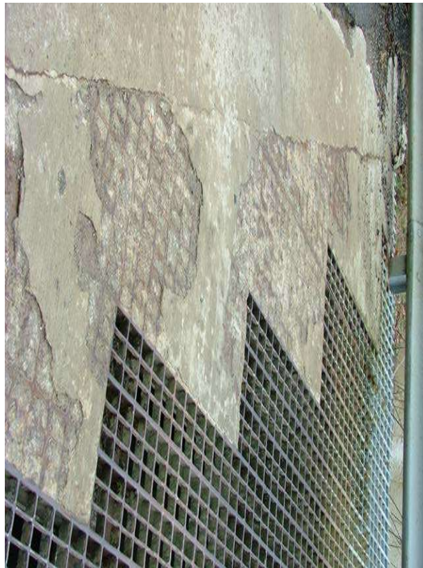
Figure 7.4.8 Filled and Un-filled Steel Grid Deck
