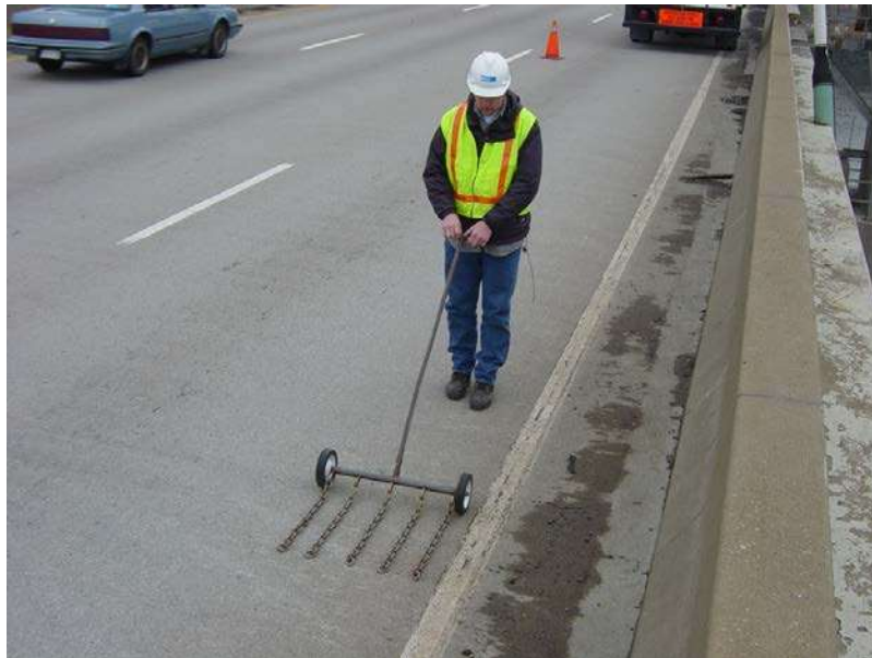
Figure 7.2.7 Sounding for Delaminated Areas of Concrete
