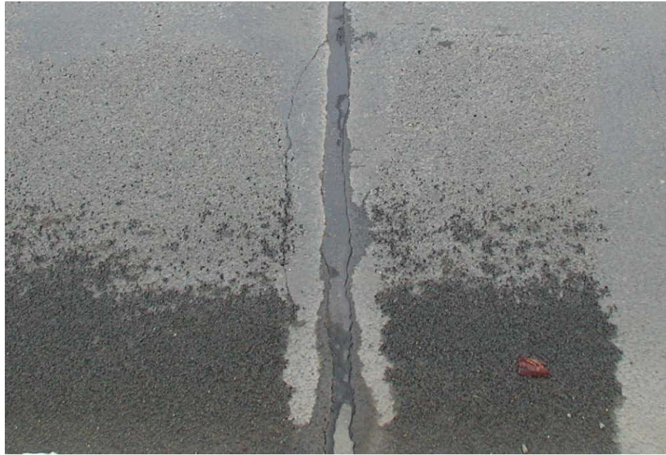
Figure 7.3.7 Deck expansion joint
